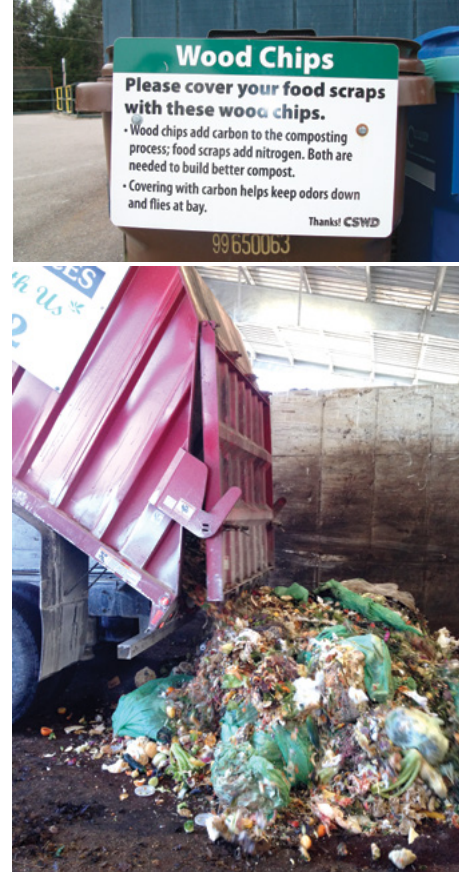
Residents using the drop-off program in Chittenden County, VT cover their food scraps with wood chips to provide carbon and to avoid odors and flies. This also helps when unloading food scraps.
