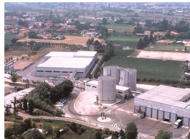
The anaerobic digestion facility in Bassano del Grappa treats separately collected residential food waste using a dry continuous flow process with three cylindrical digesters (center of photo).
