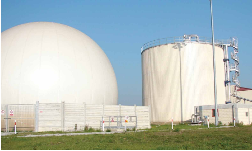
The integrated biotreatment facility in Camposampiero, which processes separately collected municipal organics, animal manure and biosolids, utilizes a two-phase wet digestion process.
