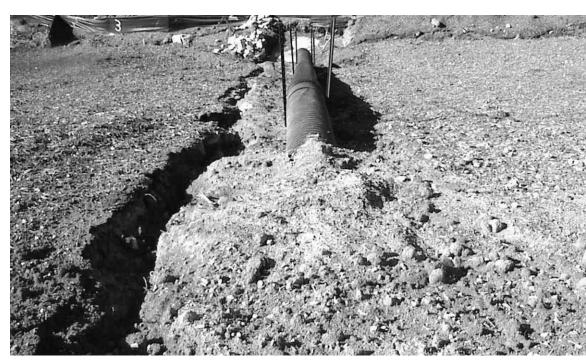
The research showed how ineffective the silt fence was in containing solids. On a 34 percent slope, total settleable and suspended solids in the water that passed through the silt fence was 32 ml/L and 26,000 ml/L, respectively versus the compost barrier (made from mixed yard trimmings) at 2.6 ml/L and 1,300 ml/L, respectively.
